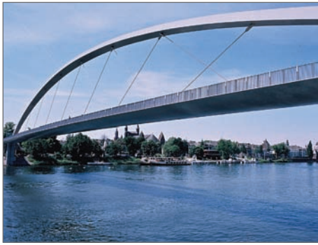
The Hoegh Brök (High Bridge) with UM in the distance.
